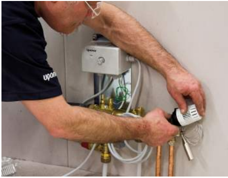
9. Montera termostatventilen.
